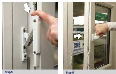
If your window has been fitted with a winkhaus restrictor to open beyond the restrictor press down (step 5). Release the catch and the window will now fully open (step 6). To close the window, push back to original position and turn the handle through 180°. Please note that a winkhaus restrictor is an optional extra and not fitted as standard.
